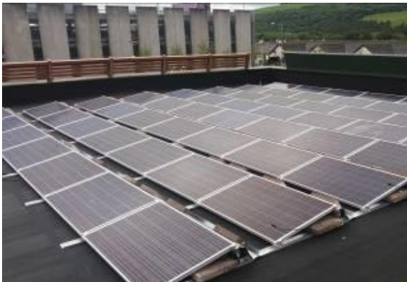
Figure 10: Flat Roof Installation
