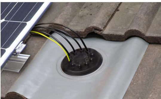
Figure 8: Dektite Solar Flashing
