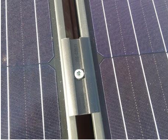
Figure 3: Module Clamps
