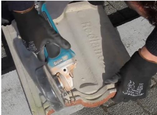
Figure 6: Tile Notching
